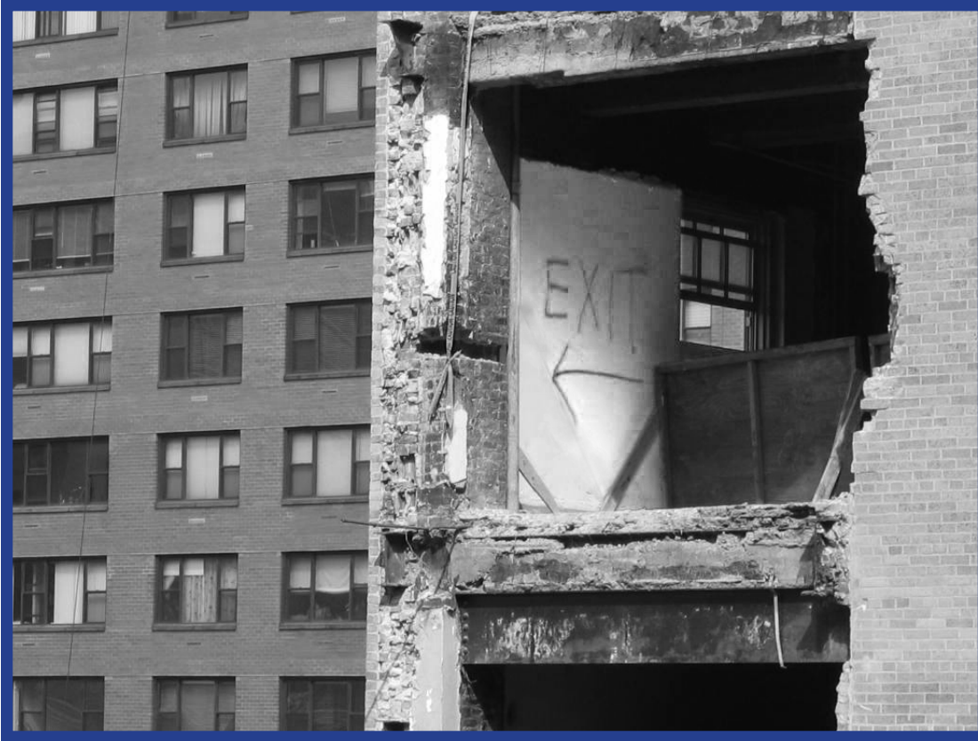
Partial building demolition provides egress shortcut.
