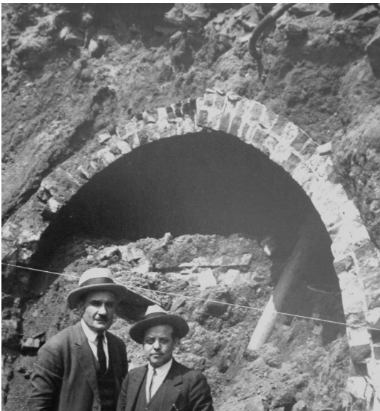
Transverse cut through typical double-wythe brick water conduit, c. 1842. Exposed in 1928 during excavations on W. 105th St.
