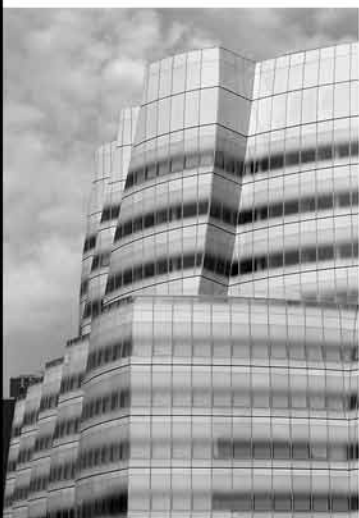
IAC Building, New York, NY
