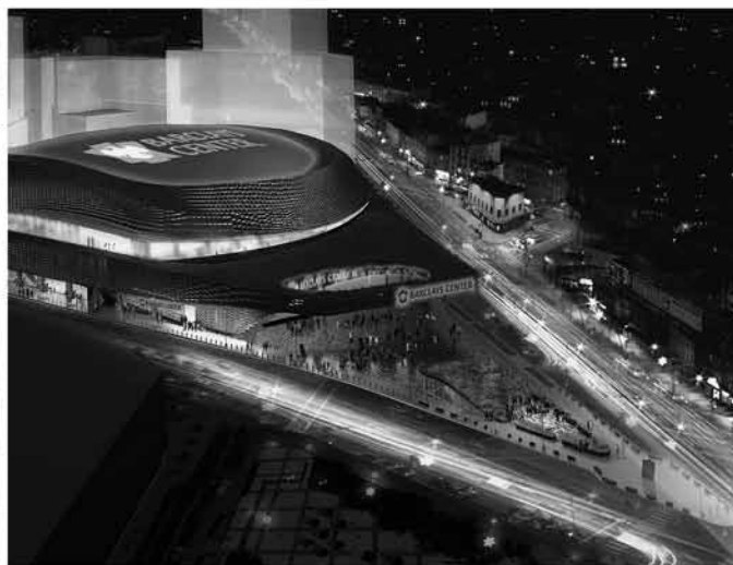
Barclays Center, Brooklyn, NY Courtesy of SHoP Architects/Ellerbe Becket
