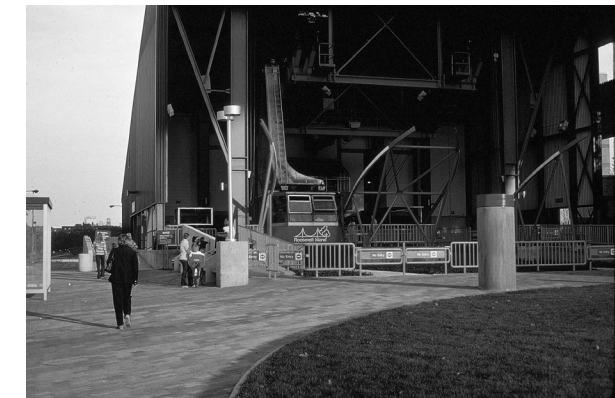
THIS PAGE, FAR LEFT The machine room of the Roosevelt Island Tram Station.
