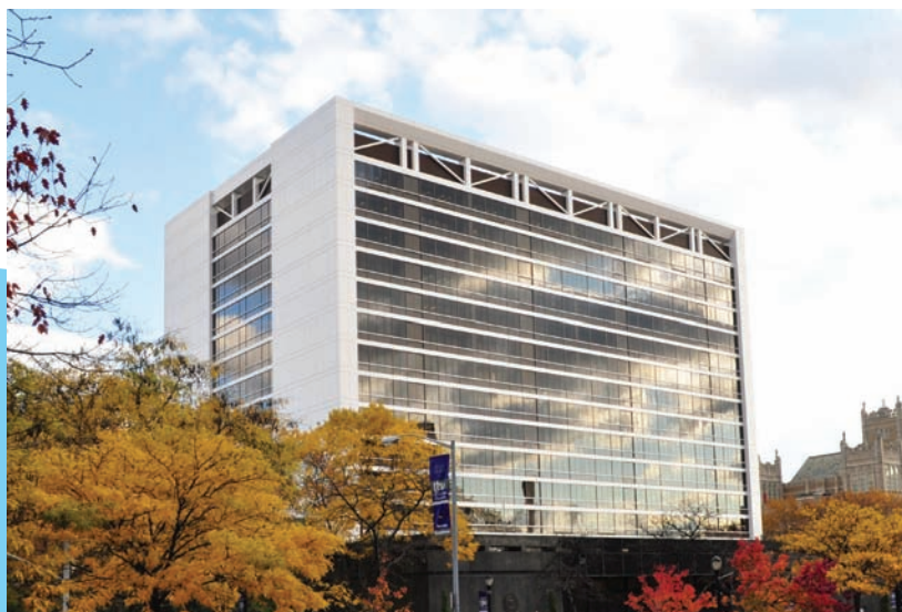
All Images: Courtesy RSD Engineering
